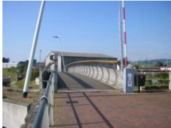
The swing bridge
