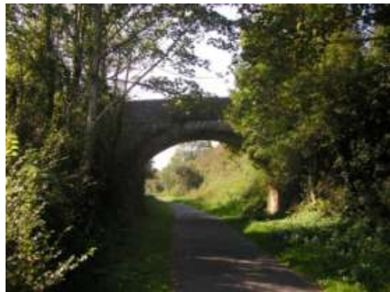
A bridge over the line
